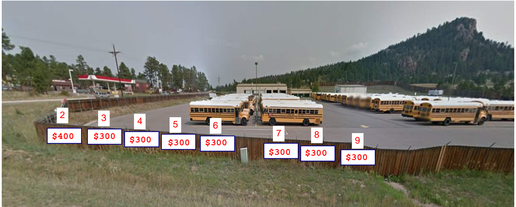
#3 - LEFT OF BUS BARN NEAR ROUND ABOUT - VISIBLE FROM CHURCH ACROSS N. TURKEY CREEK
